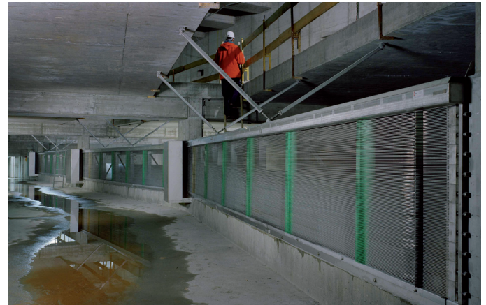
Installation of 3 CSO screens at the inflow channel of Geneva's WWTP
