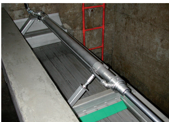
ROMAG CSO screen RSU. Relief end with hydraulic cylinder and cleaning carriage. Concrete sill forms the emergency relief.
