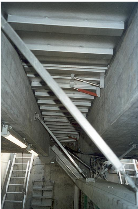
Neuhof Baar: Flood relief and storage channel Accessible cover with folding rails (small cover on the left).
