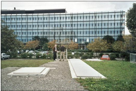
Neuhof Baar: Flood relief and storage channel Accessible cover with folding rails (small cover on the left).
